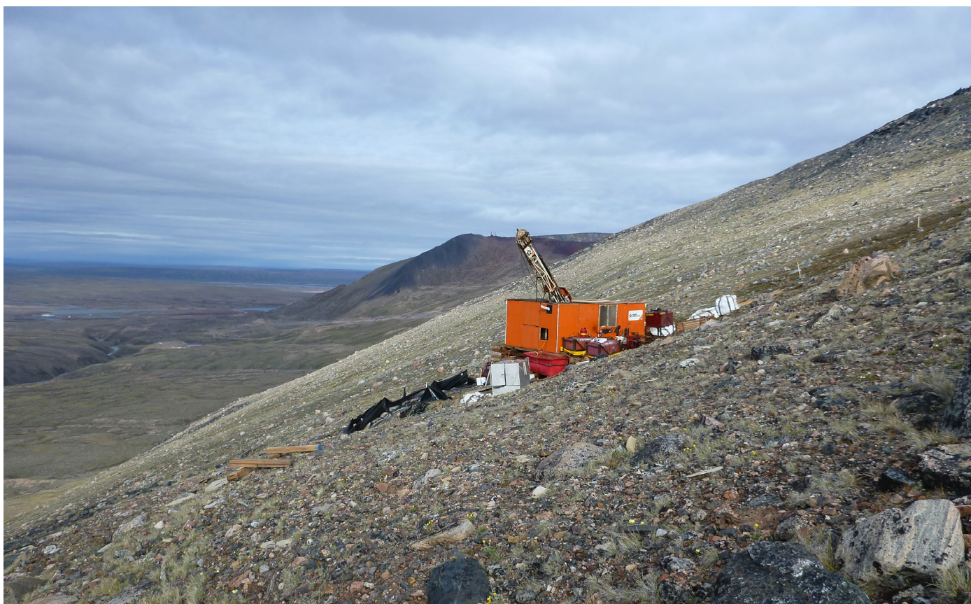
Exploration drilling at Deposit No 2, with view of Deposit No 1 in the background, Mary River project. Courtesy of BIMC
