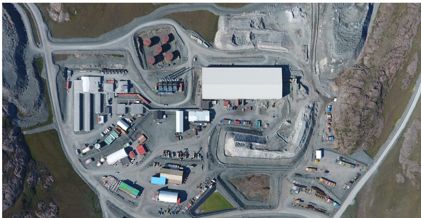
Aerial view directly overhead the Doris camp and mine infrastructure, TMAC's Hope Bay mine. Courtesy of TMAC Resources Inc
