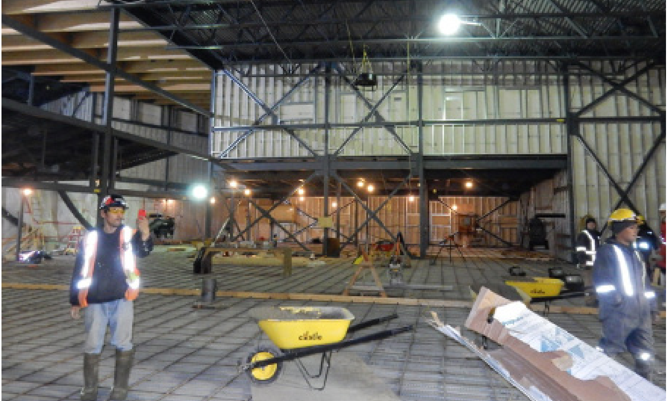
Construction of Tuugaalik High School in Naujaat.
