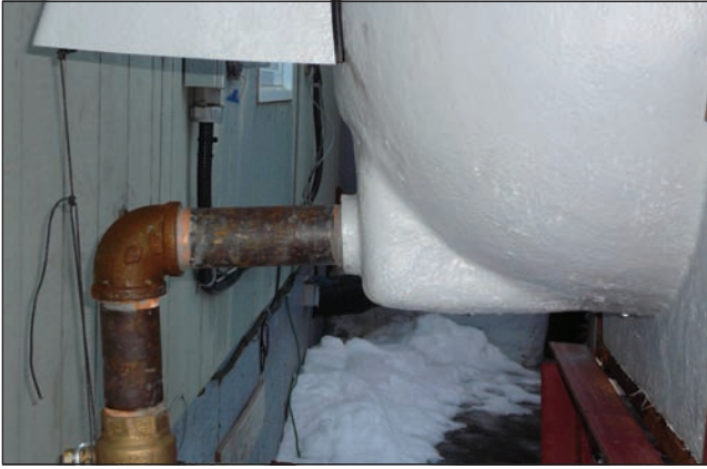
6.2a End-wall feed configuration
