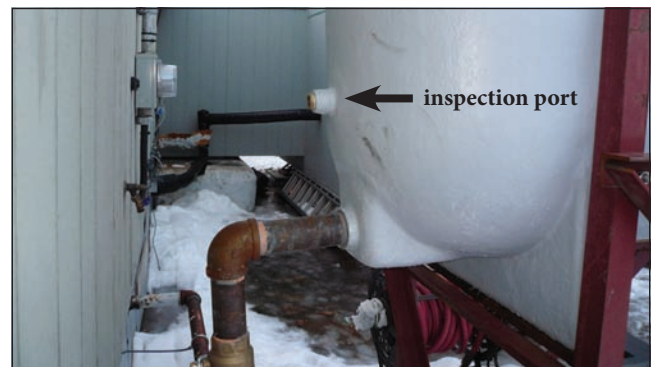
5.3b Inspection port on a double-wall fibreglass tank
