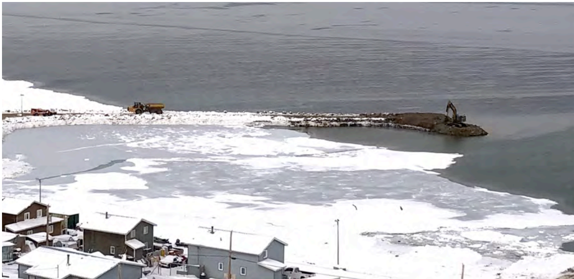
Start of Breakwater construction at Pond Inlet. Photograph Courtesy of Advisian
