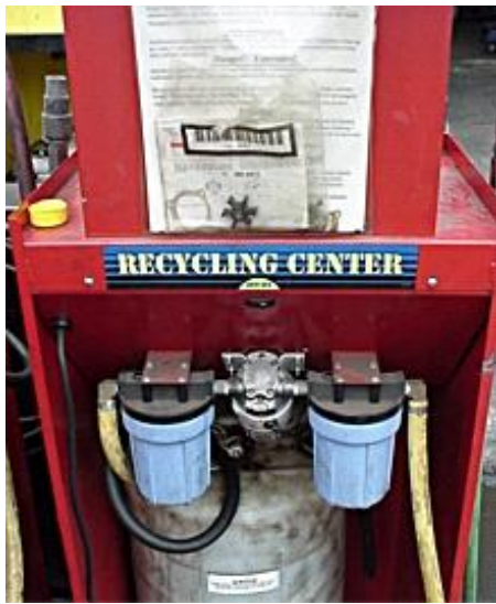
Figure 2 – Typical Antifreeze Recycling System
