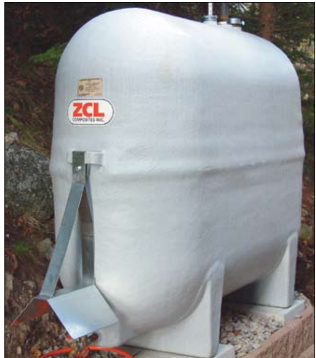
5.4 Fibreglass, 1,135 litre (250 gallon) Atauhittuktuk ukhukyuakakvik. Nalungilutit munagitjutait kaangani ukhukyuat amangutait (piksaliukhimayuk ZCL Composites, Edmonton, AB).
