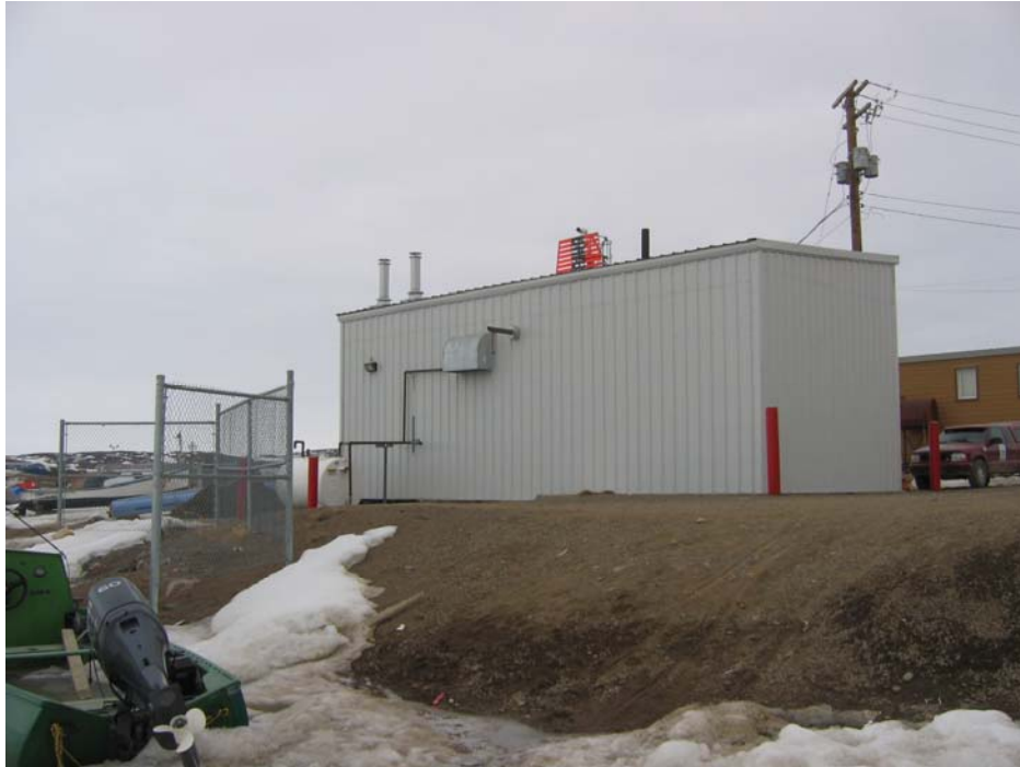
Figure 2: City of Iqaluit, Lift Station #1
